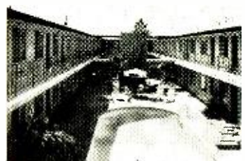
APARTMENT—48 Outlets—Two Antennas (24 Outlets each)—No Amplification: The Paramount Riviera—12447 Paramount Blvd., Downey, California.
